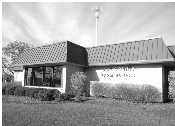
The east facing doors were replaced by a window when the KCFB entrance was moved to the north side of the building during renovations in 1984. A mansard roof was added.
